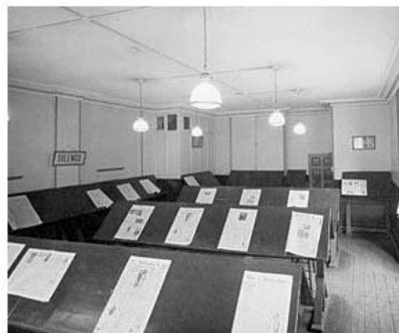
The Reading Rooms
